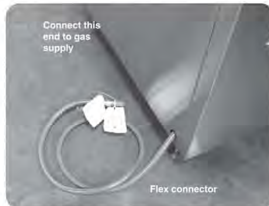
Fig. 7-2 - Natural gas outdoor connector
