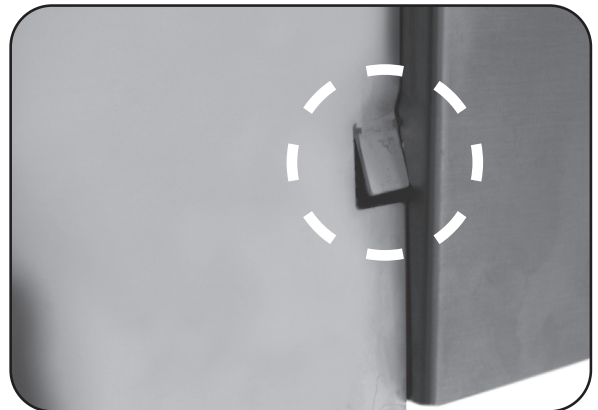
Fig. 26-3 Tab slightly bent in for clearance
